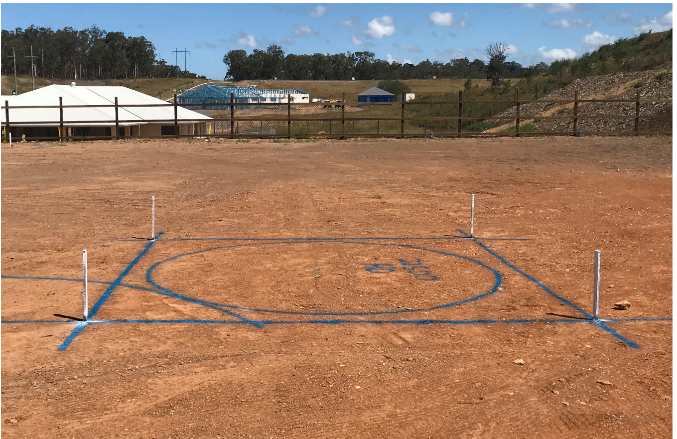
Rainwater Tank Ground Mark out
