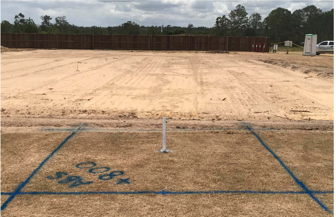
Secondary Wastewater Treatment System Tank Ground Mark out
